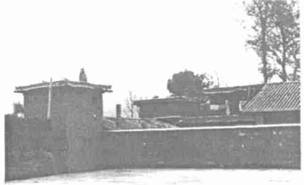
Fig.9 The perimeter walls around the piazza
