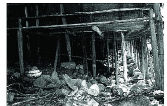
图3 千脚落地屋的柱脚 Fig.3 Thousand Feet House's foot falling to the ground
