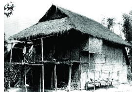
图2 德宏傣族竹楼 Fig.2 Dehong Dai bunch of bamboo building
