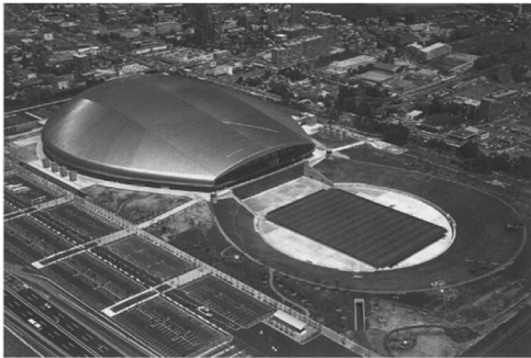
图5 札幌穹顶鸟瞰 Fig.5 Bird's eye view of Sapporo Dome
